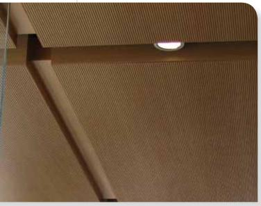
The ACGI Encore™ System combines superior acoustical performance with the aesthetic quality of wood.
